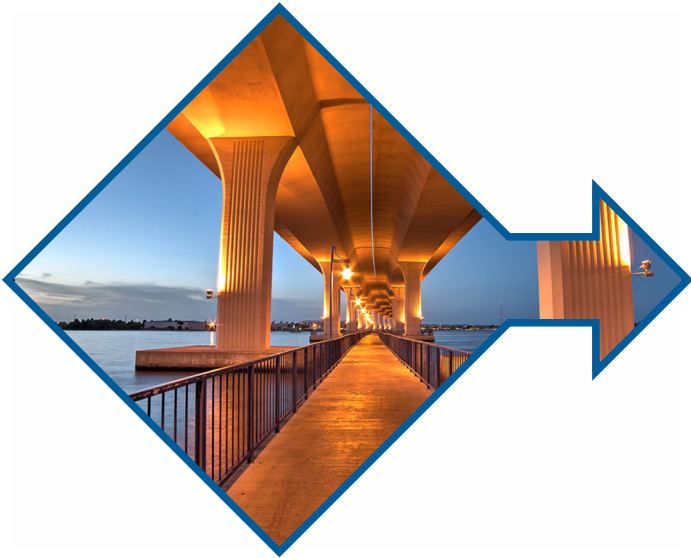
STRUCTURAL HEALTH MONITORING
